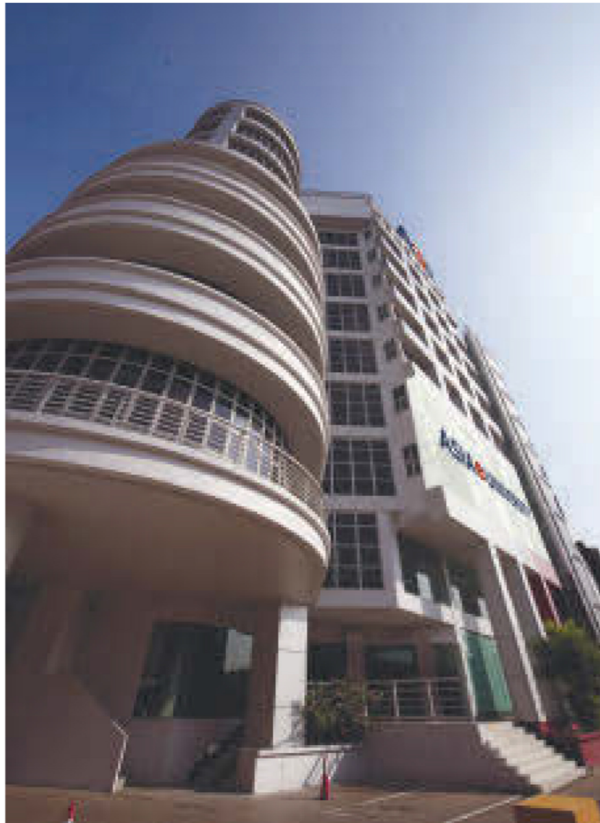
AeU's new relocated Subang Jaya campus.
